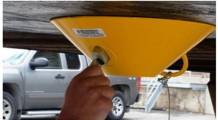
4. Remove allen key, insert Medeco cylinder. Make sure the cylinder is oriented correctly.
